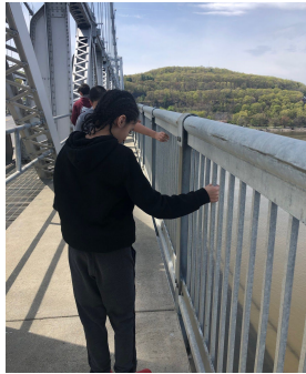
Jacob testing out the bridge's vibrations.
